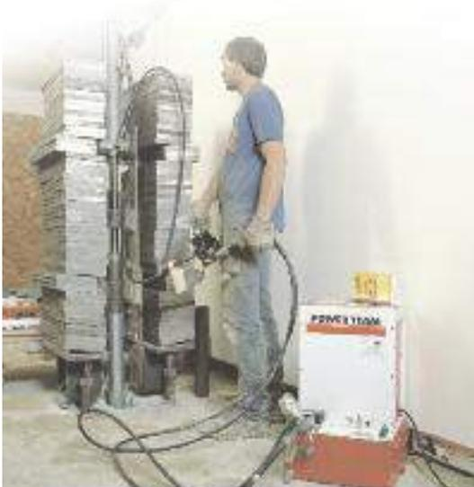
PQ- series pump used to drive piers to lift and stabilize building foundation.
